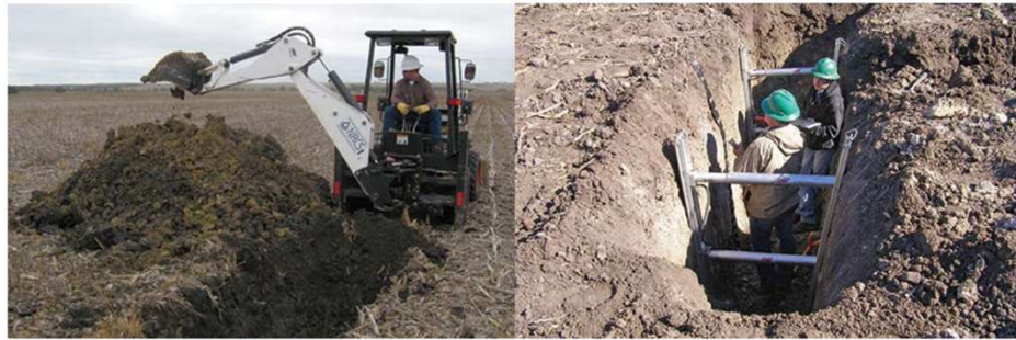
Figure 2: A backhoe excavation and safety measures in deep trenches.
